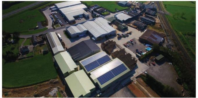
Solar Electric Ireland won the project with a design for 250kWp or 960 modules set out on the east-west facing roofs of the cold-storage facility. The modules were mounted on an existing building and a new building constructed in the summer of 2015.
